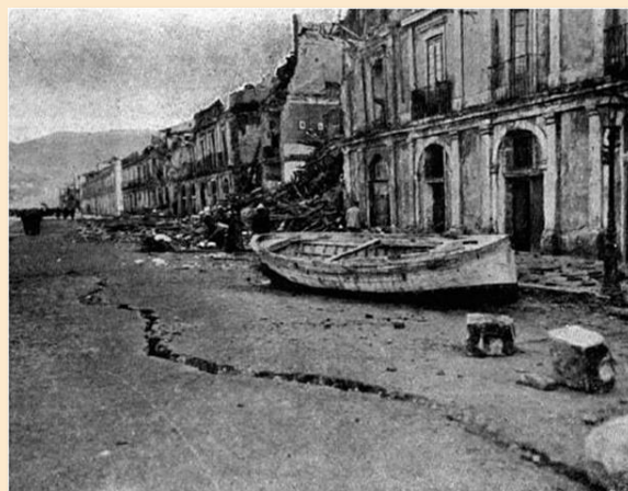
Damages of the 1908 earthquake and tsunami in Messina, Italy (photo from the INGV photo gallery http://www.ingv.it/ufficio-stampa/stampa-e-comunicazione/Galleria-immagini/archivio-immagini-terremoti/photo_album.2010-04-28.5890391000/ ).
